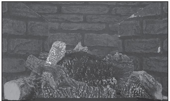
Figure 11.9 Install Left Top Log
