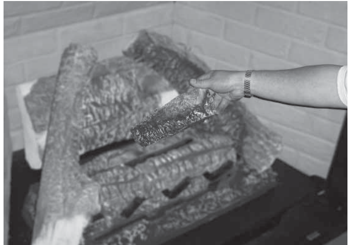
Figure 15.15 Positioning Right Middle Log
