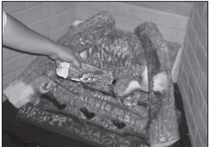
Figure 15.16 Positioning Left Middle Log
