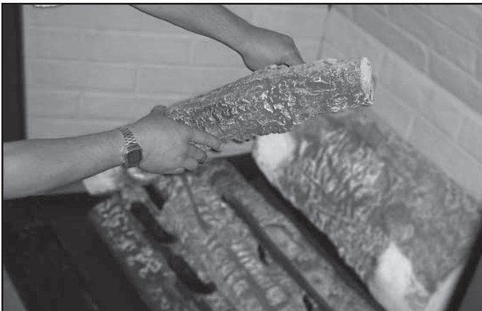
Figure 15.13 Positioning Left Log
