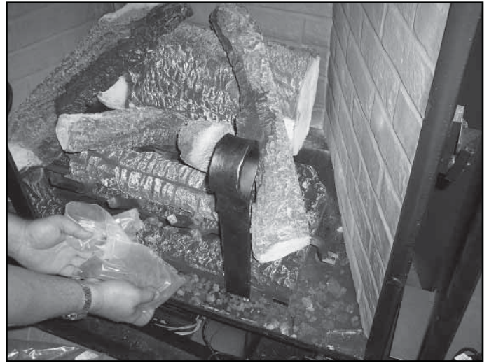
Figure 15.19 Placing Lava Rock
