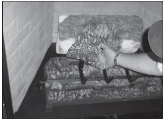
Figure 15.11 Positioning Left Front Log
