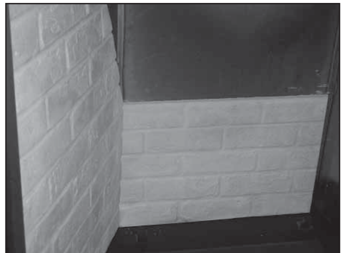
Figure 15.3 Install Lower Back Refractory
