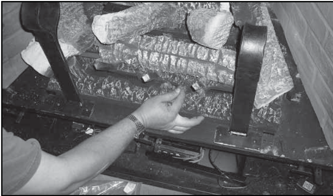
Figure 15.17 Placing Rockwool
