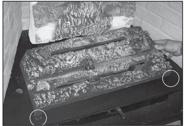
Figure 15.9 Positioning Ember Bed
