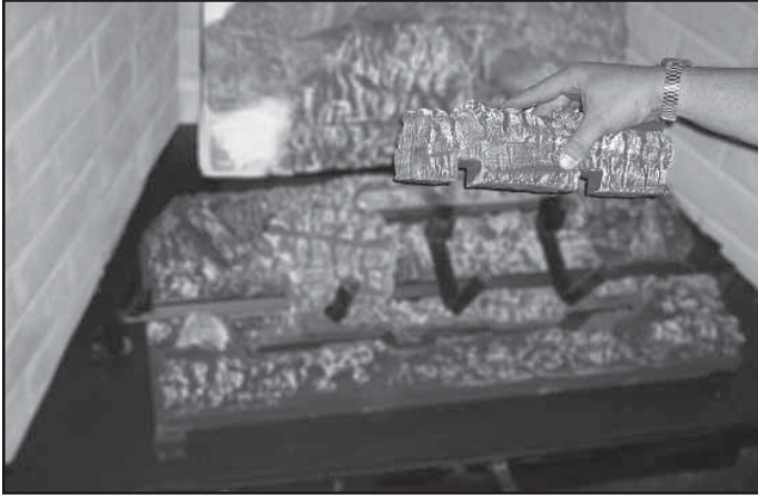
Figure 15.12 Positioning Right Front Log
