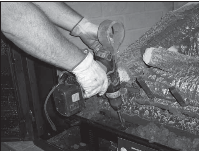
Figure 15.18 Installing Andirons
