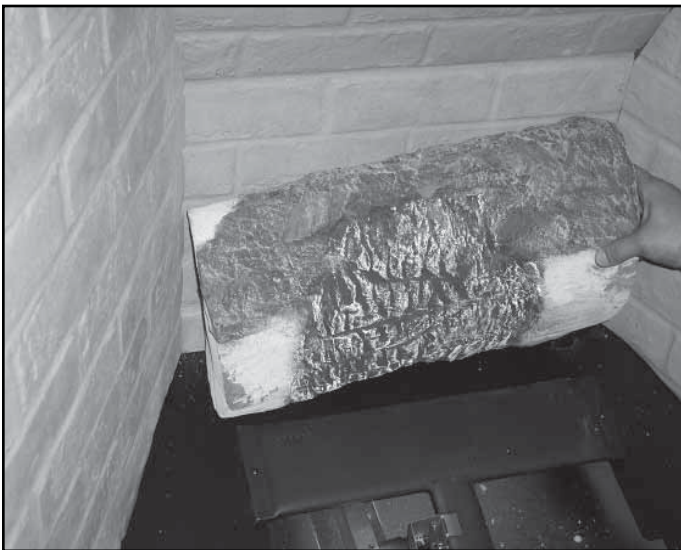
Figure 15.8 Positioning Rear Log
