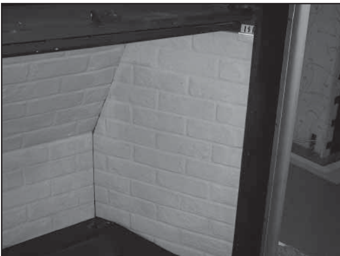
Figure 15.5 Install Right Side Refractory
