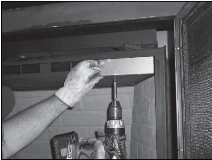
Figure 15.7 Adjust the Vertical Baffle
