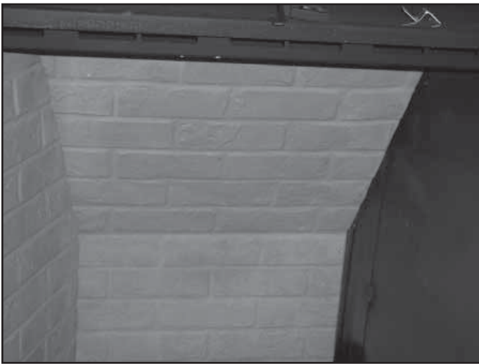
Figure 15.4 Install Upper Back Refractory
