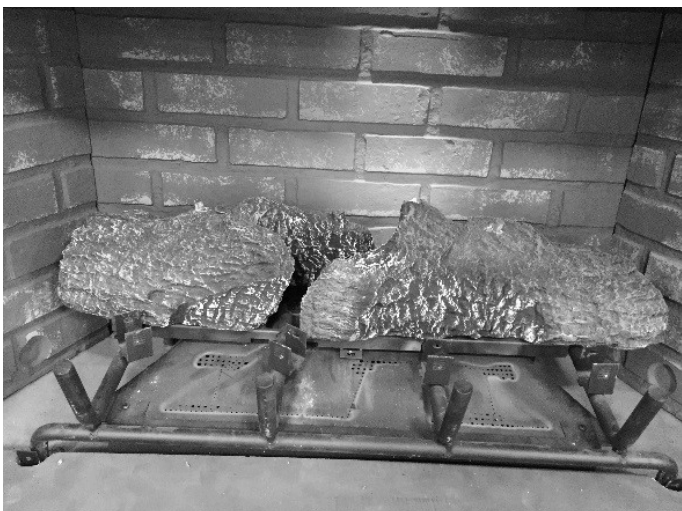
Figure 14.8 Left and Right Rear Log Placement
