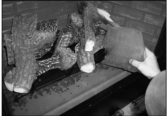
Figure 14.21 Placement of Lava Rock
