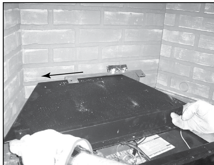
Figure 14.30 Side Burner Assembly to Left
