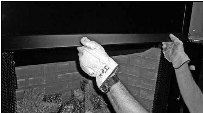
Figure 14.27 Installing the Hood
