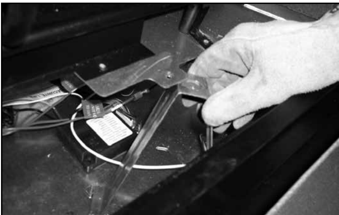
Figure 14.3 Rotate Support
