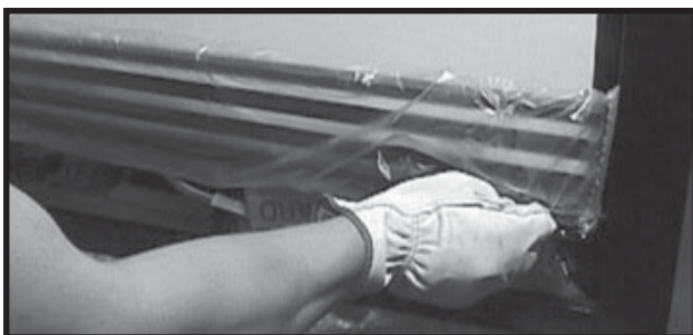
Figure 13 - Control Access Panel Removal
