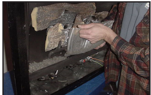
Figure 15 - Placing the Lava Rock
