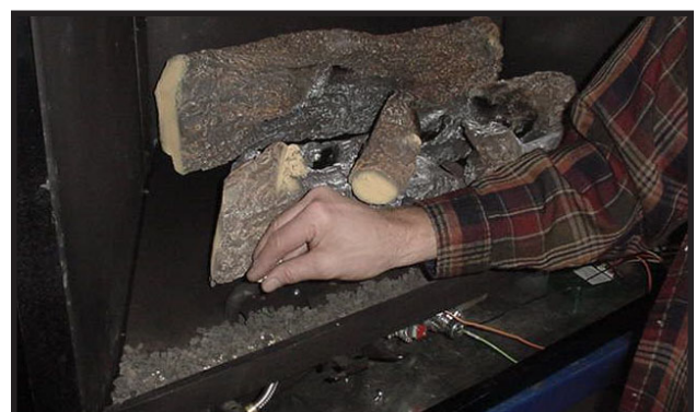
Figure 16 - Placing the Vermiculite
