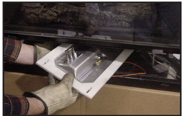
Figure 20 - Removing the Valve Assembly
