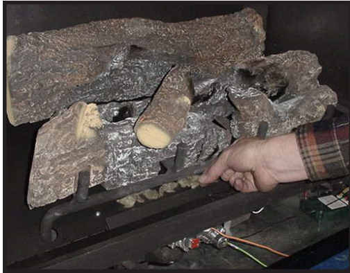
Figure 17 - Placing the Rock Wool
