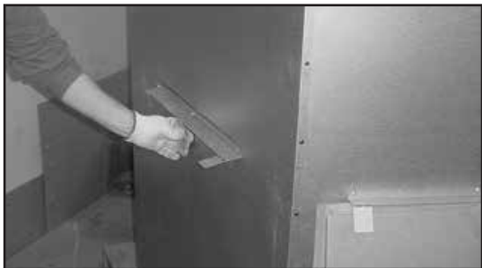
Figure 3.7 Bend Refractory Brackets Back Down
