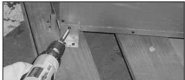
Figure 3.11 Removing Shipping Brackets
