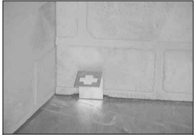
Figure 8.8 Grate Retaining Bracket in Place
