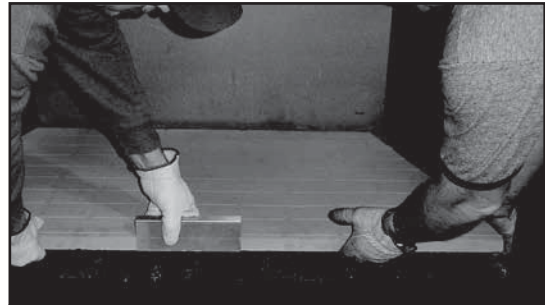
Figure 3.10 Lifting Out Hearth Stone
