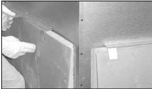
Figure 3.6 Unpack Back Refractory
