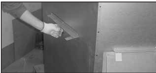
Figure 3.7 Bending Refractory Shipping Tabs Back Down
