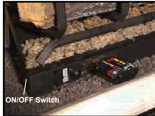
Figure 15 - Battery Replacement
