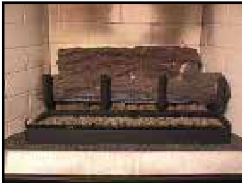
Figure 10 - Placing the Front Log
