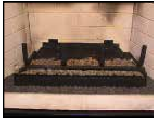
Figure 7 - Rock Wool Placement
