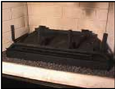
Figure 6 - Placing the Grate Assembly
