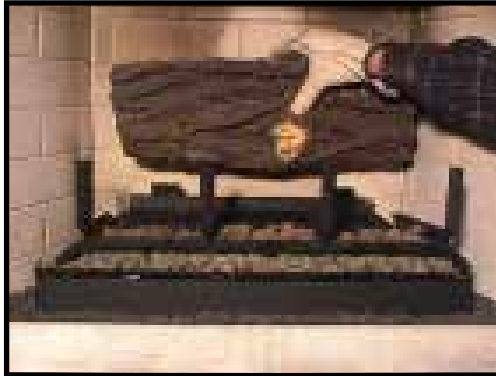
Figure 9 - Rear Log Placement
