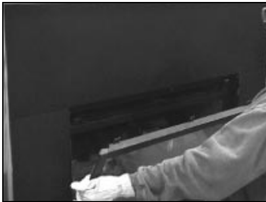
D - Removing the Glass to be Cleaned
