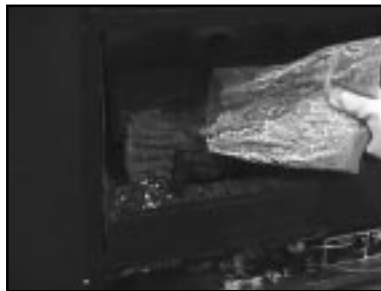
Figure 23 Placing the Vermiculite
