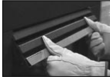
Figure 17 Installing the Upper Grille
