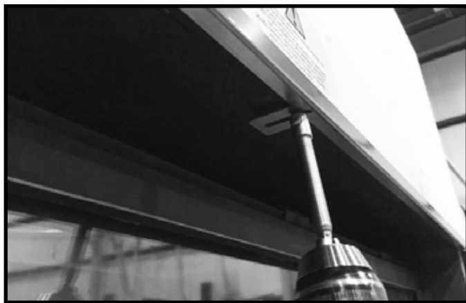
Figure 10.5 Install Trim Ring
