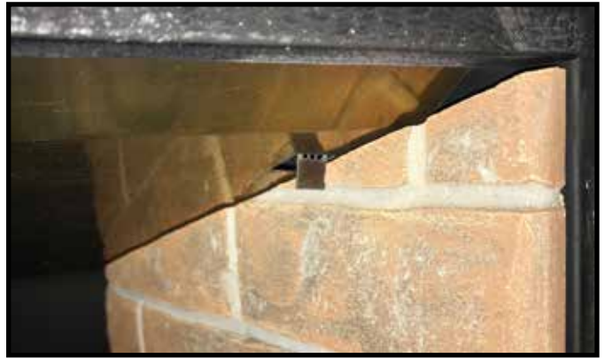
Figure 7 Right Refractory Handbend Tab
