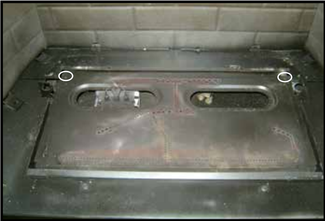
Figure 4.9 Remove Screws from Burner Assembly Rear Corners
