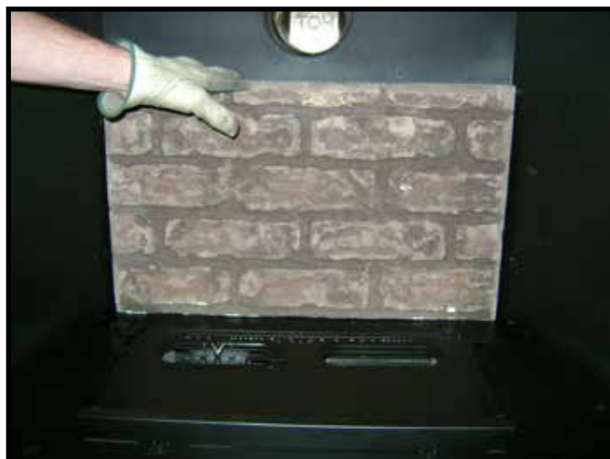
Figure 4.5 Back Refractory Removal
