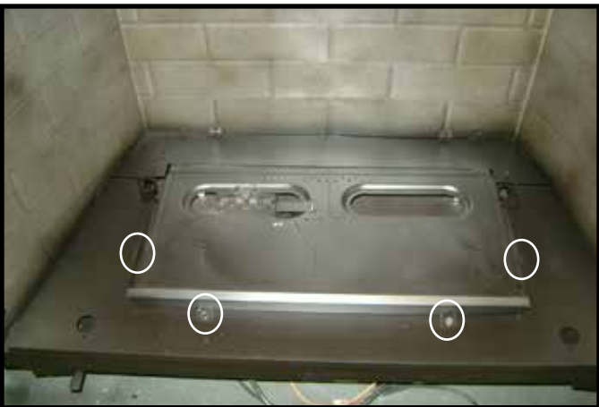
Figure 4.10 Remove Burner Skirt
