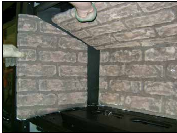
Figure 4.3 Top Refractory Removal
