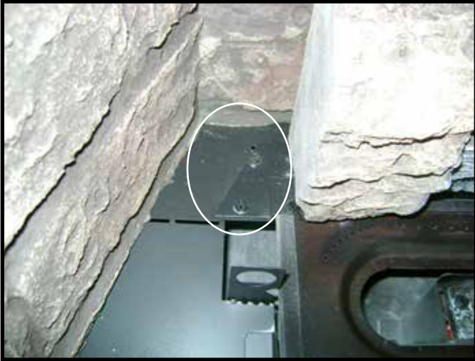
Figure 4.8 Remove Screws from Log Tabs
