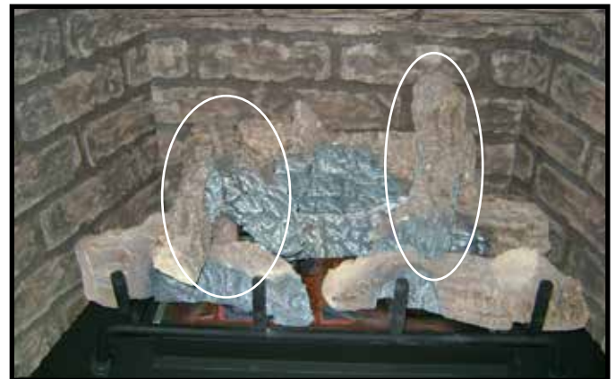
Figure 4.6 Remove Top Two Logs
