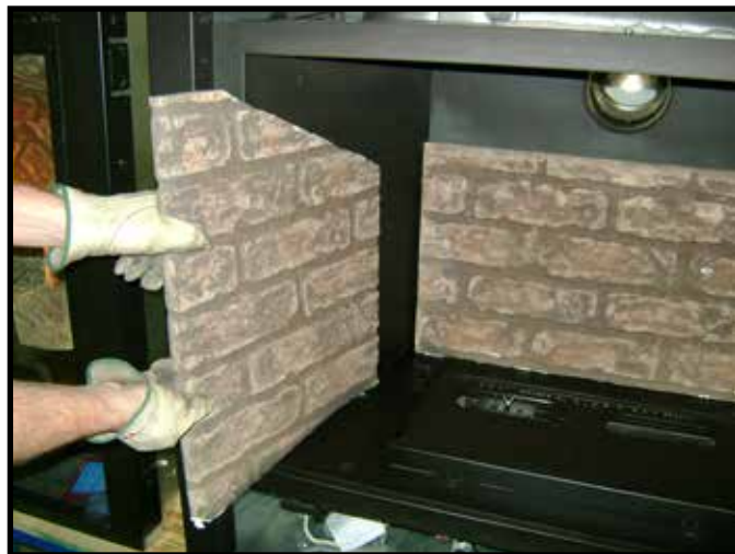
Figure 4.4 Side Refractory Removal
