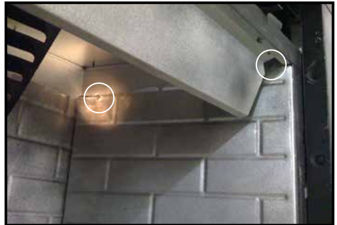
Figure 4.7 Top Screws For Metal Refractory
