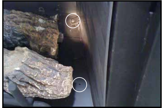
Figure 4.6 Bottom Screws For Metal Refractory
