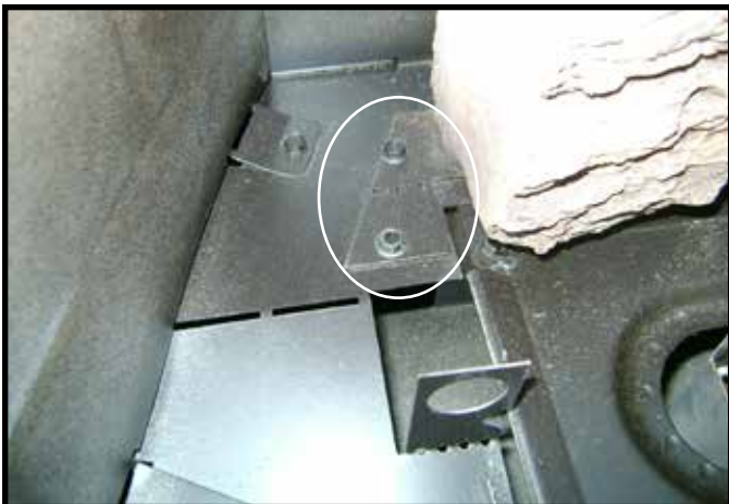
Figure 4.5 Remove Screws from Log Tabs
