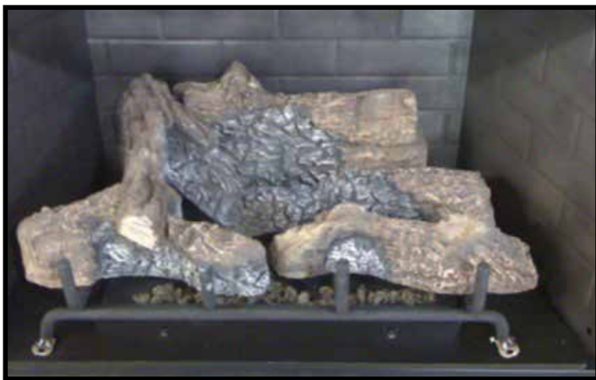
Figure 5. Left Log in Proper Position
