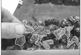
Figure 8.11 Place individual pieces of embers in front of and around the gas log where they can be seen. Space them so
