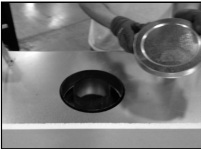
Figure 6.2 Remove the seal cap. (Generic Fireplace Shown)
