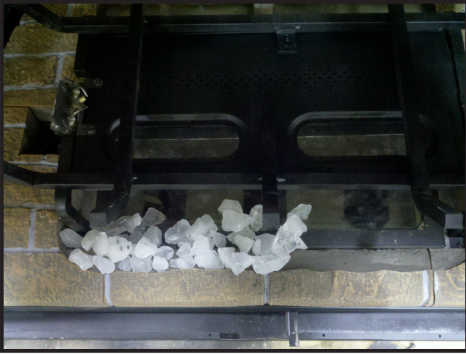
Figure 11.19. Install Teco-Sil
