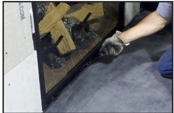
Figure 11.8. Securing Bottom Glass Clips
