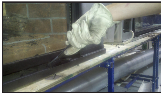
Figure 11.3. Inserting Glass Clip Tool
