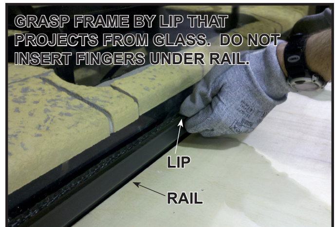
Figure 11.6. Installing Glass
