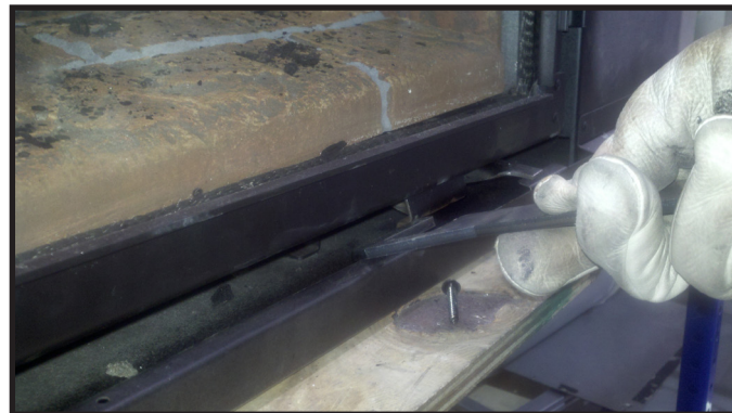
Figure 11.2. Glass Clip Tool Location
