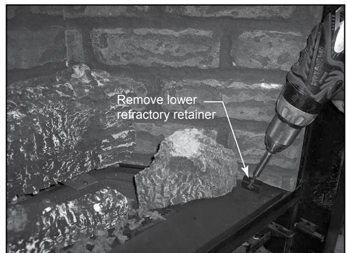
Figure 4.17 Remove Refractory Retainer
