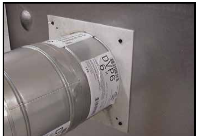
Figure 6.12 (Generic Fireplace Shown) Attach the first vent section (it will snap into place). Slide the insulation gasket onto the vent section, up against the appliance and over the tabs. Use two self-tapping screws to secure gasket to outer wrap.
