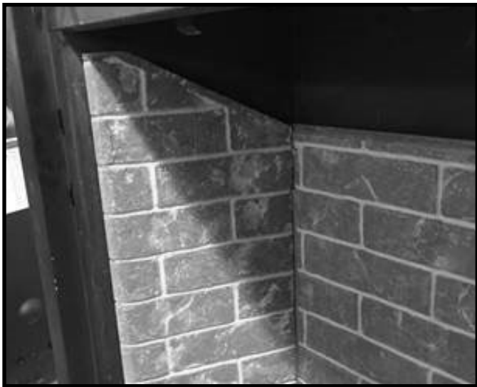
Figure 11.4 Install Left Refractory Panel
