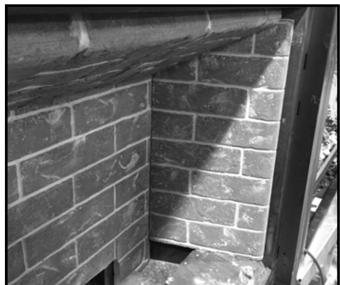
Figure 11.7 Right Refractory Panel Installed
