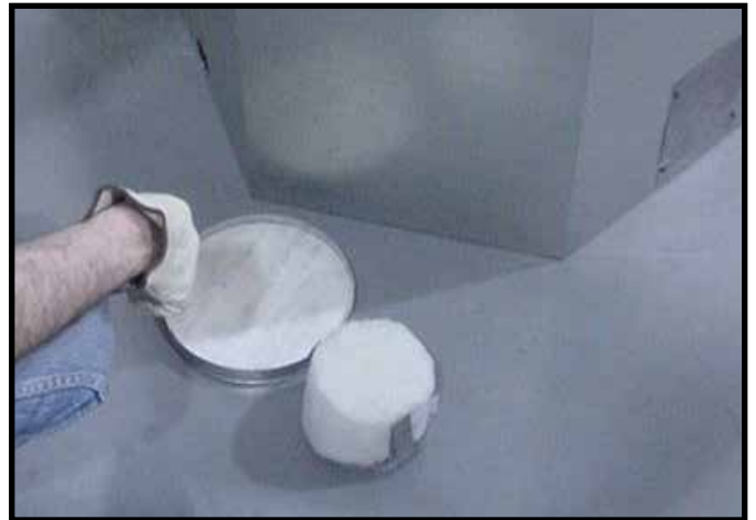
Figure 6.11 (Generic Fireplace Shown) Discard the seal cap, remove and discard the insulation basket. Note: Once the seal cap has been removed it CANNOT be reattached.
