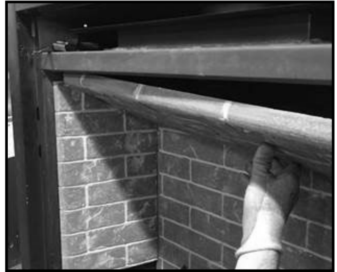
Figure 11.5 Install Top Refractory Panel
