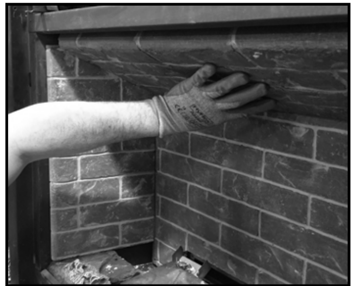
Figure 11.6 Install Right Refractory Panel
