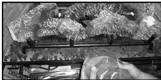
Figure 14.3 Placement of Lava Rock
