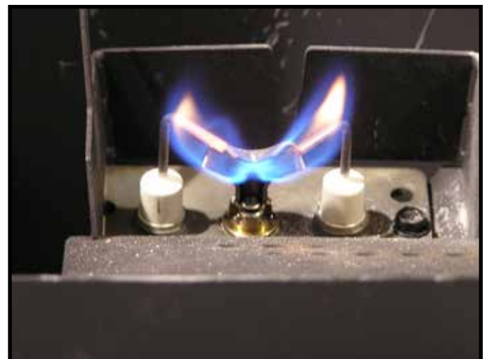
Figure 3.1 IPI Pilot Flame Patterns
