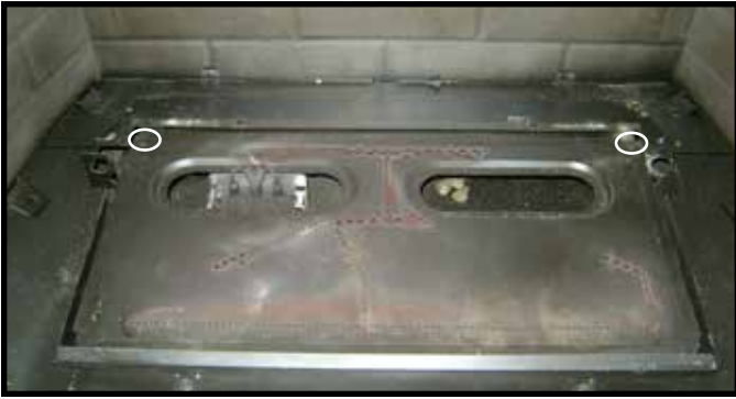
Figure 3.8 Remove Screws from Burner Assembly Rear Corners
