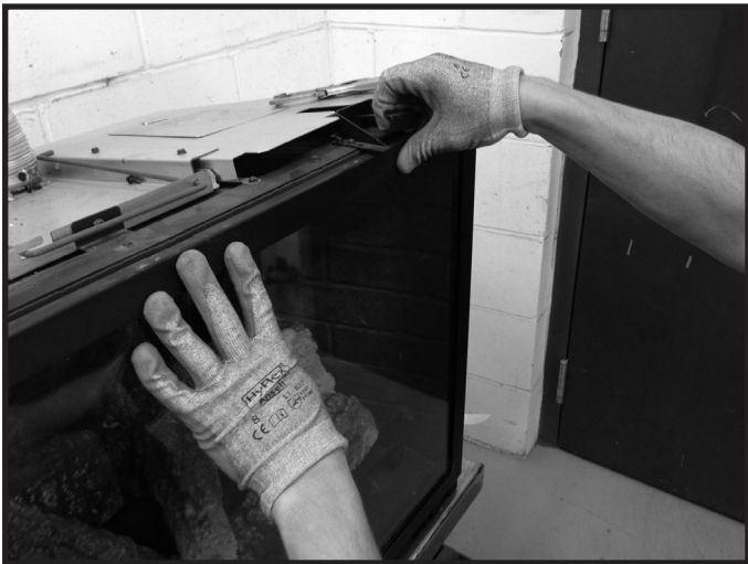
Figure 4.3 Release Glass Latches One at a Time
