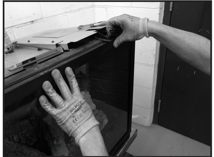
Figure 11.3 Release Glass Latches One at a Time
