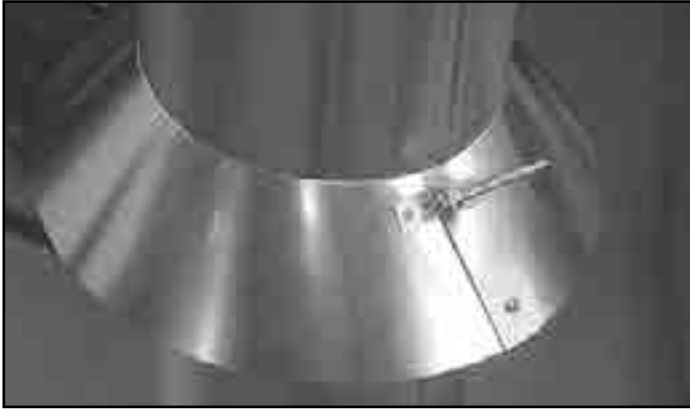
Figure 7.14 Insert Bolt into Brackets
