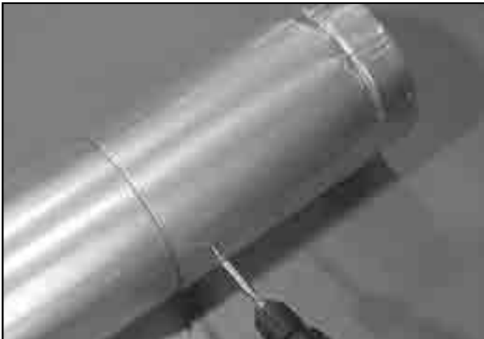
Figure 7.4 Screws into Slip Section
