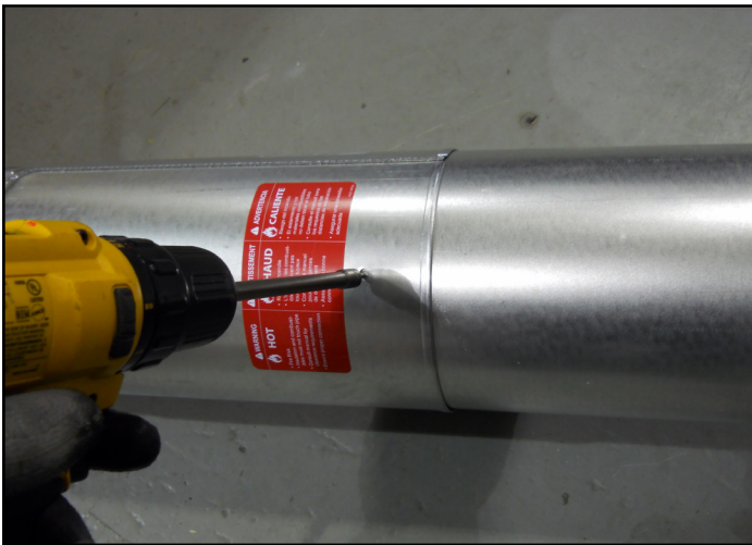
Figure 7.4 - Screws into Slip Section
