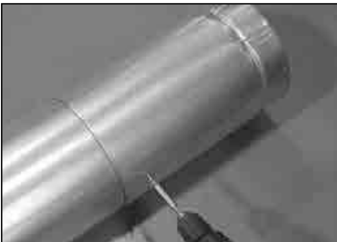
Figure 7.4 Screws into Slip Section
