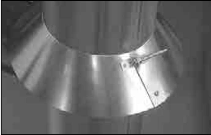
Figure 7.14 Insert Bolt into Brackets
