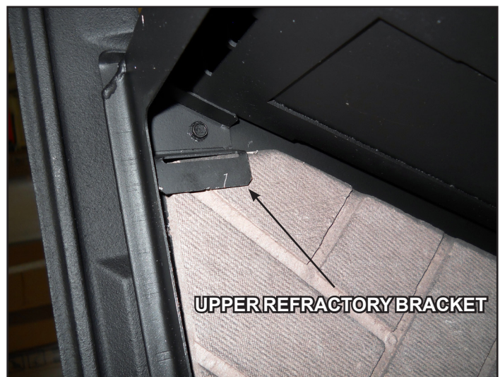
Figure 10.7 - Upper Refractory Brackets
