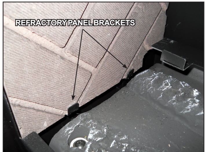
Figure 10.6 - Bottom Refractory Brackets
