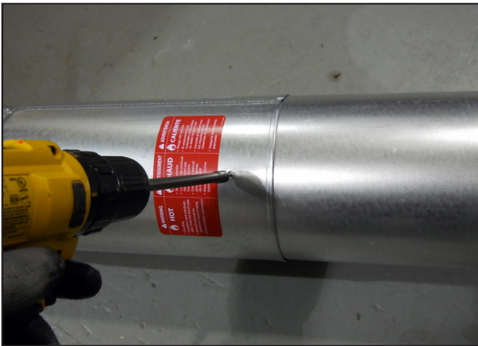
Figure 7.4 - Screws into Slip Section
