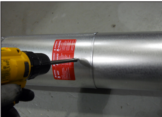
Figure 7.4 - Screws into Slip Section
