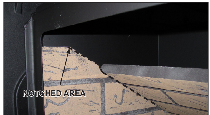
Figure 10.7 - Place Top Refractory
