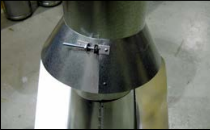
Figure 7.14 - Insert Bolt into Brackets
