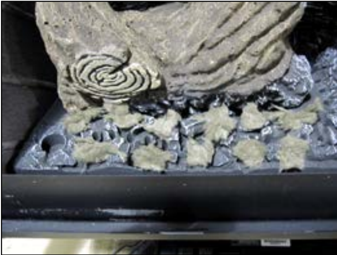
Figure 10.13 - Place Mineral Wool
