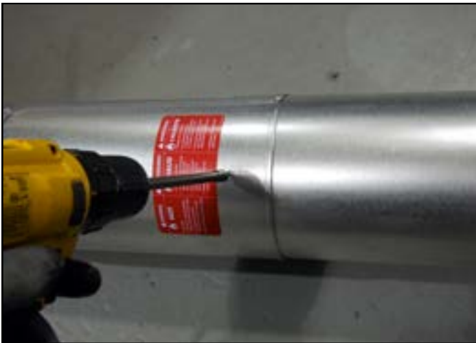
Figure 7.4 - Screws into Slip Section
