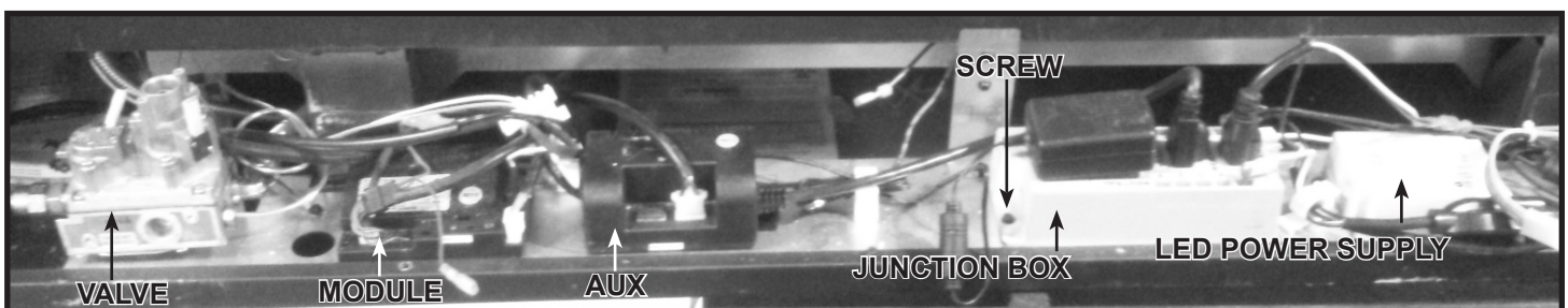
Figure 8.4 Valve Cavity (Lower Access Cover Panel Removed)
