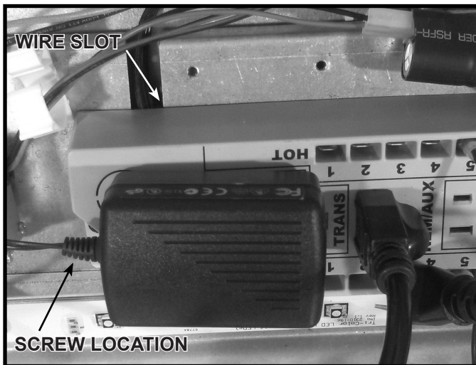
Figure 8.3 Junction Box Detail
