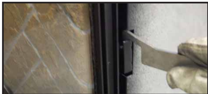
Figure 11.7. Fasten Side Glass Clips
