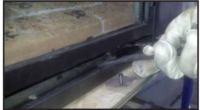
Figure 11.2 Glass Clip Tool Location
