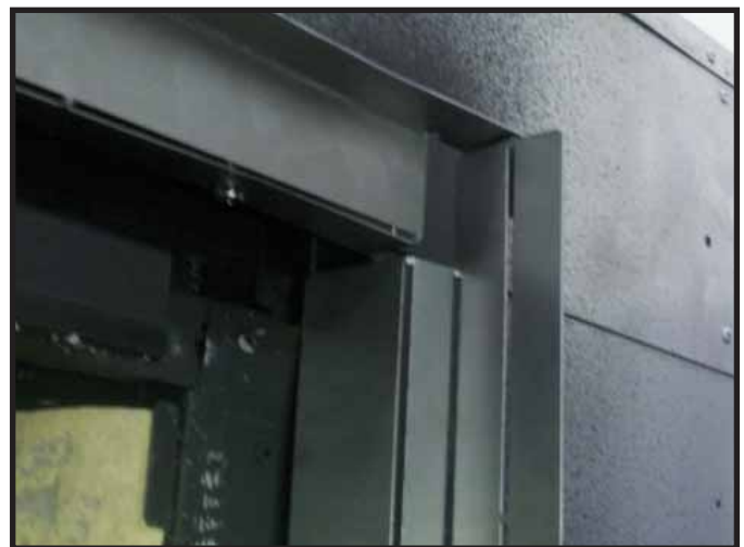
Figure 10.4 Top/Side Finishing Templates Installed
