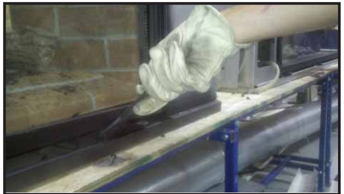
Figure 11.3 Inserting Glass Clip Tool
