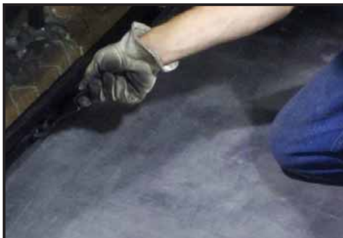
Figure 11.8. Fasten Lower Glass Clips
