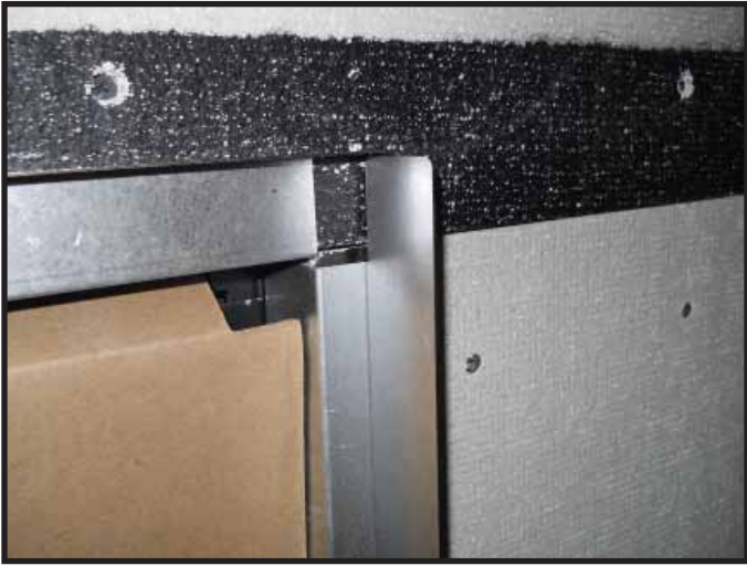
Figure 10.5 Finishing Template Bends
