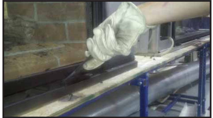
Figure 11.3. Inserting Glass Clip Tool
