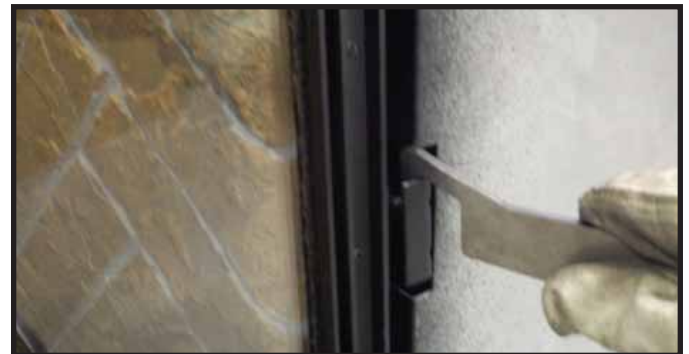
Figure 11.7. Securing Side Glass Clips
