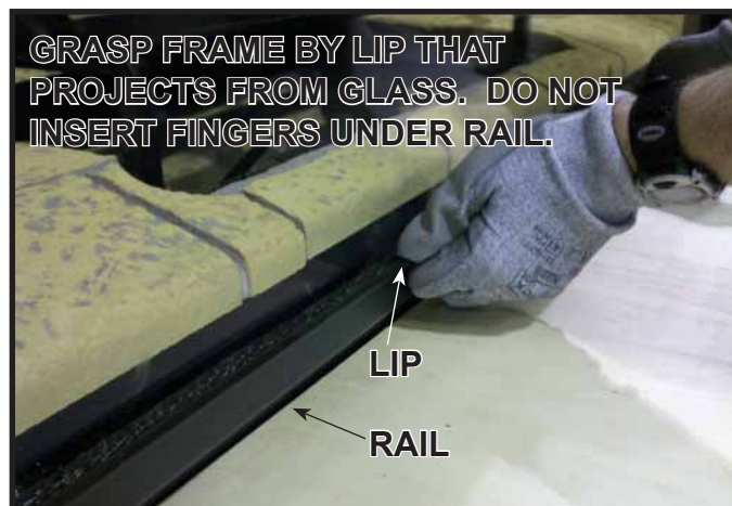
Figure 11.6. Installing Glass
