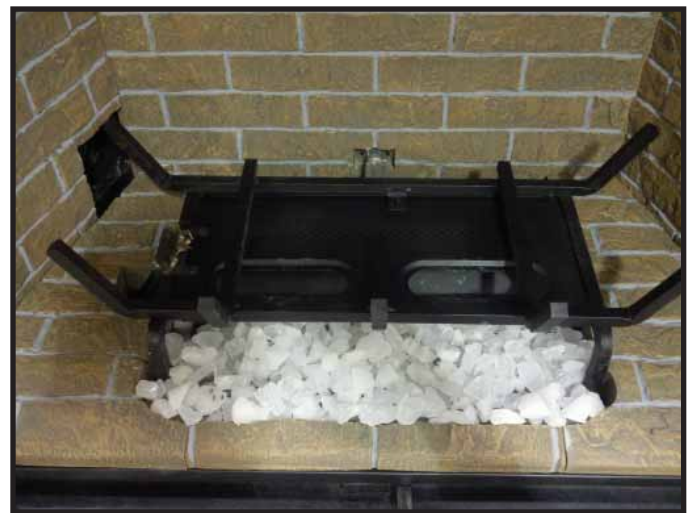
Figure 11.9. Ember Glass Area Covered with Teco-Sil
