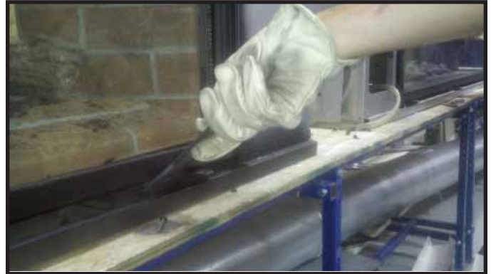
Figure 11.3. Inserting Glass Clip Tool
