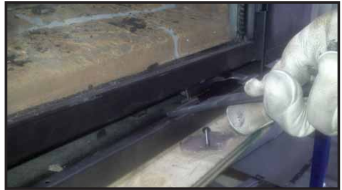
Figure 11.2. Glass Clip Tool Location
