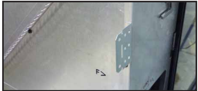
Figure 6.4 Nailing Tab Bent Out for Installation
