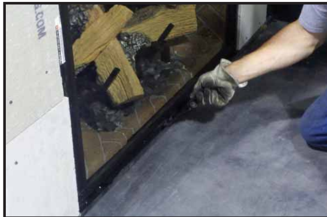
Figure 11.8. Securing Bottom Glass Clips
