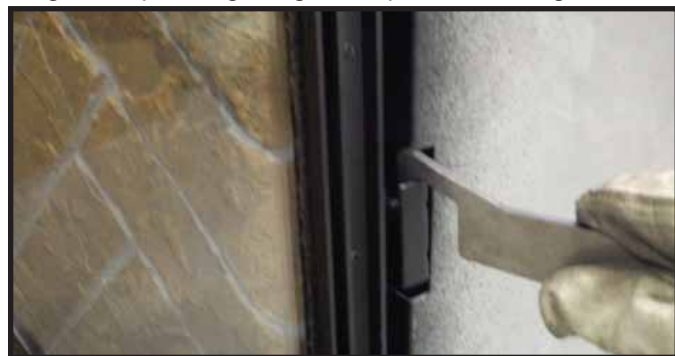
Figure 11.7. Securing Side Glass Clips
