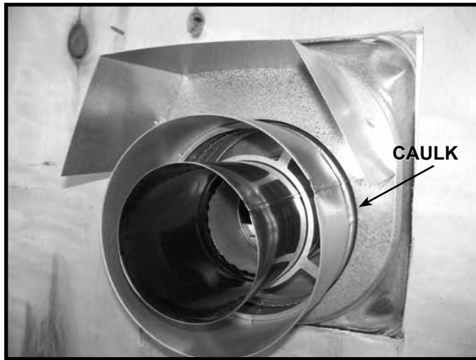
Figure 6.1. Firestop - Exterior View
