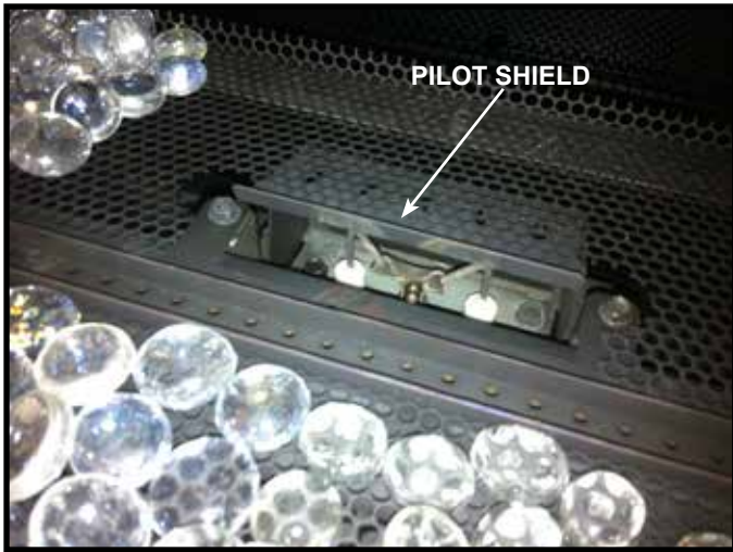
Figure 14.3. Placing Glass Rock Media on Pilot Shield
