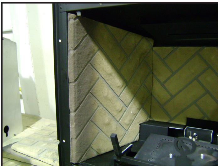
Figure 3. Install Side Refractory
