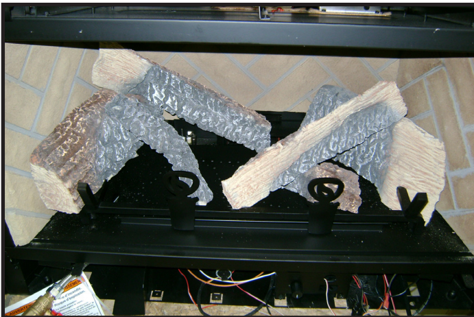
Figure 2. Refractory and Logs Installed
