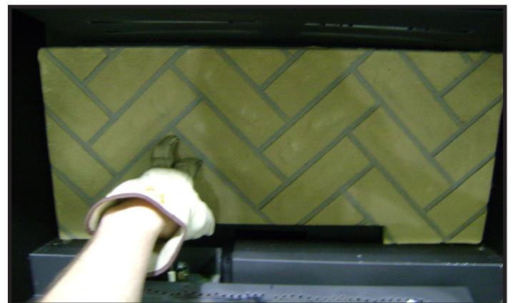
Figure 2. Install Back Refractory
