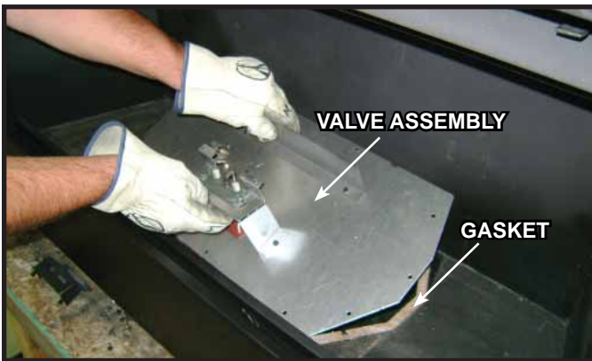
Figure 16.6 Remove Valve Plate
