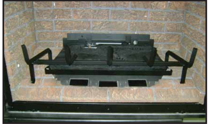
Figure 6. Front Base Refractory Installed
