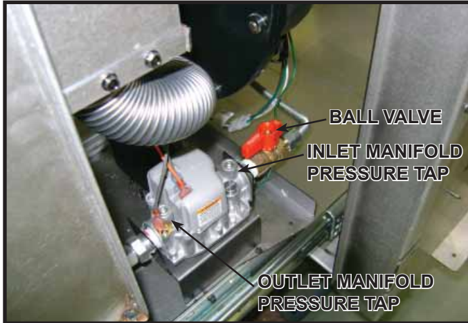
Figure 13.1 Location of Gas Ball Valve
