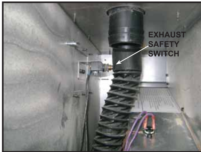
Figure 14.3 Exhaust Safety Switch
