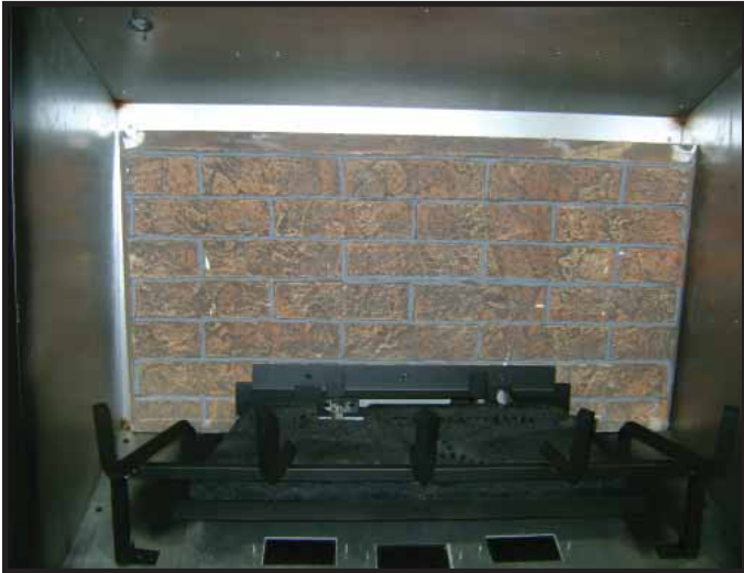
Figure 1. Rear Refractory Installation
