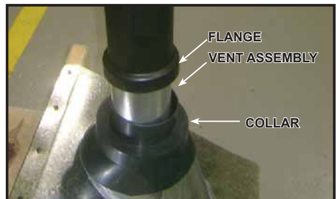
Figure 10.11 Vent Flange Installed on Storm Collar
