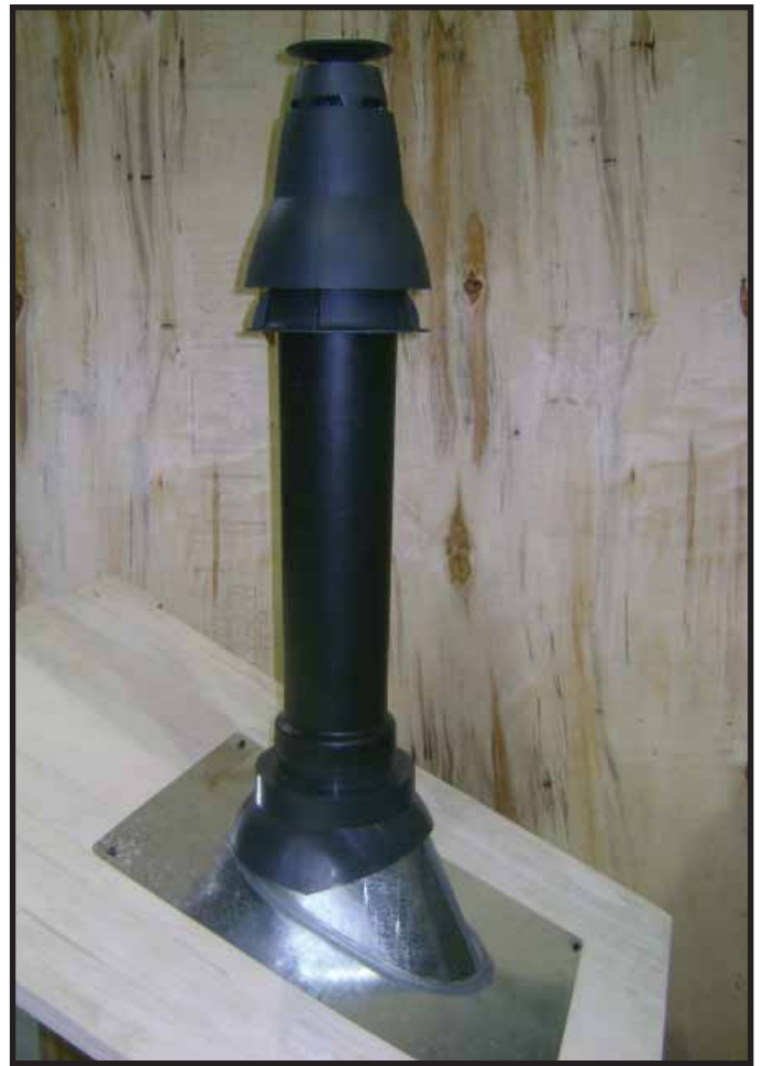
Figure 10.14 Correct Vertical Termination Installation
