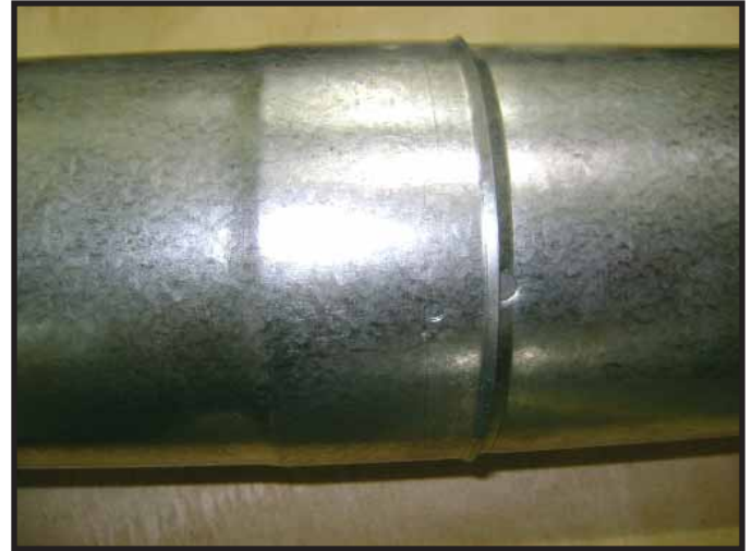
Figure 10.7 Securing Horizontal Pipe Sections
