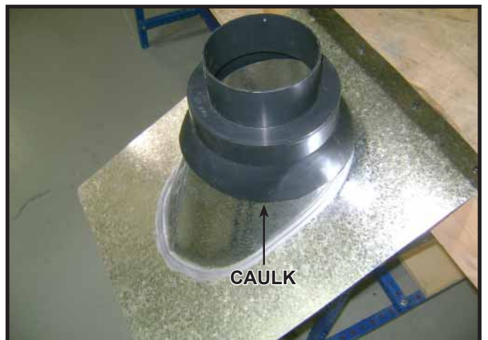
Figure 10.10 Caulk Around Metal/Plastic Seam
