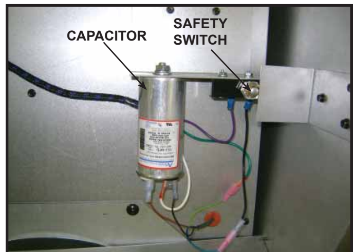
Figure 14.6 Capacitor and Safety Switch
