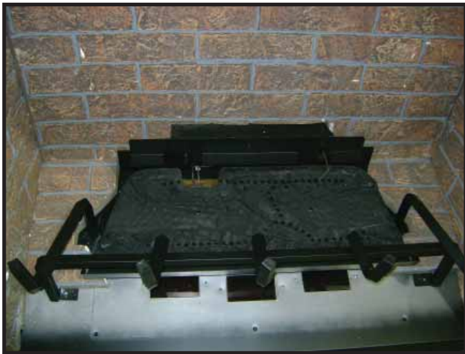
Figure 5. Left and Right Base Refractory Installed
