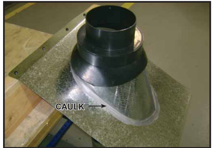
Figure 10.9 Caulk Around Flashing
