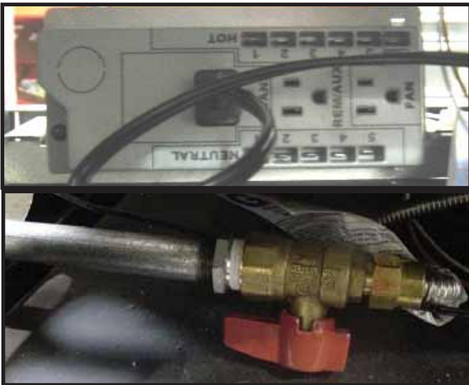
Figure 13.1 Preparation to Install Splatter Guard
