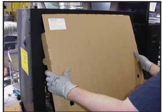
Figure 13.4 Installation of Splatter Guard
