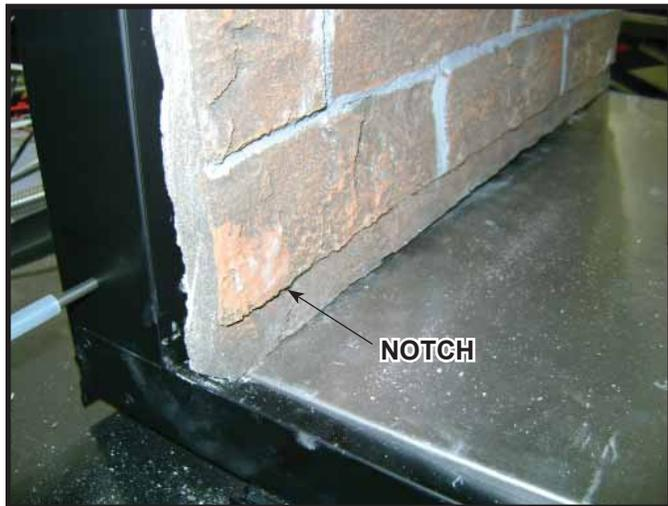
Figure 14.14 Notched End of Side Refractory
