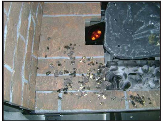
Figure 14.22 Ember Placement on Base Refractory
