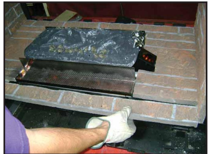
Figure 14.18 Positioning Outer Bottom Refractory.
