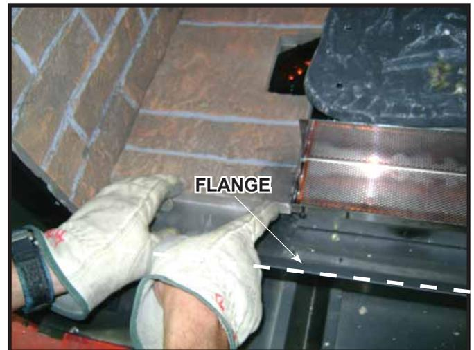
Figure 14.17 Positioning Left and Right Middle Base Refractory
