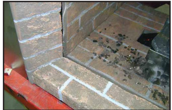
Figure 14.27 Outer Hearth Installation
