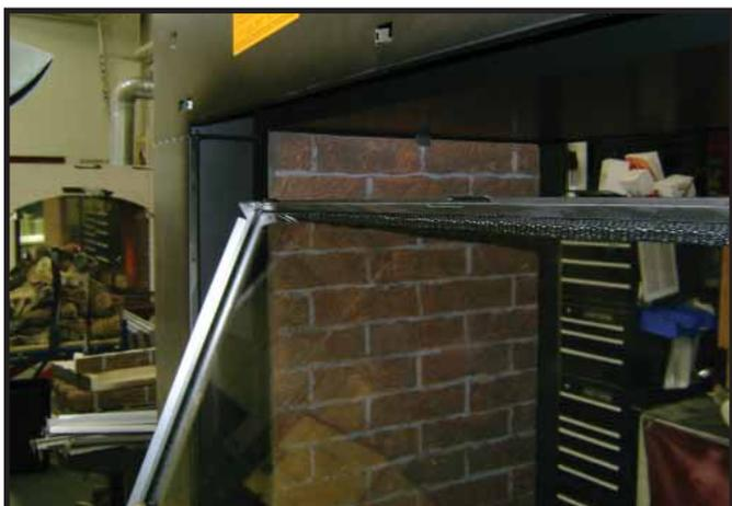
Figure 14.2 Initial Positioning of Frame into Opening.
