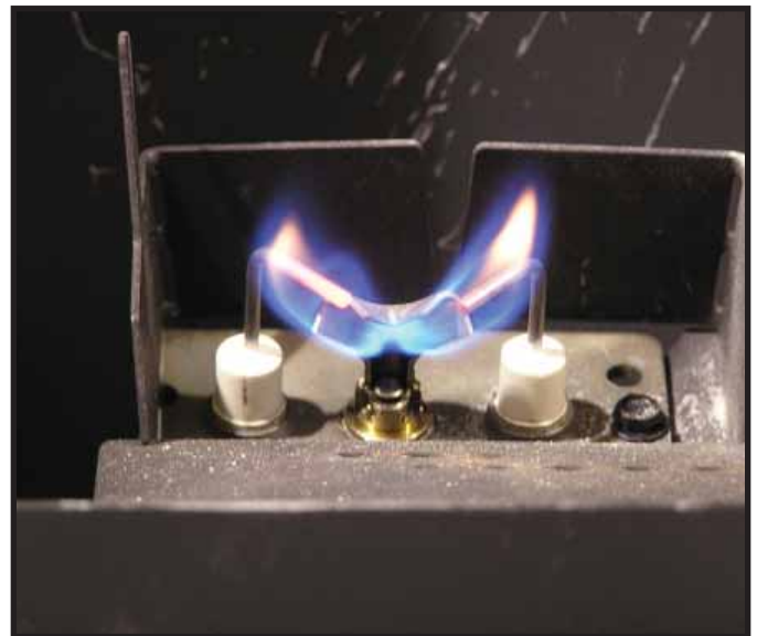
Figure 3.1 IPI Pilot Flame Patterns
