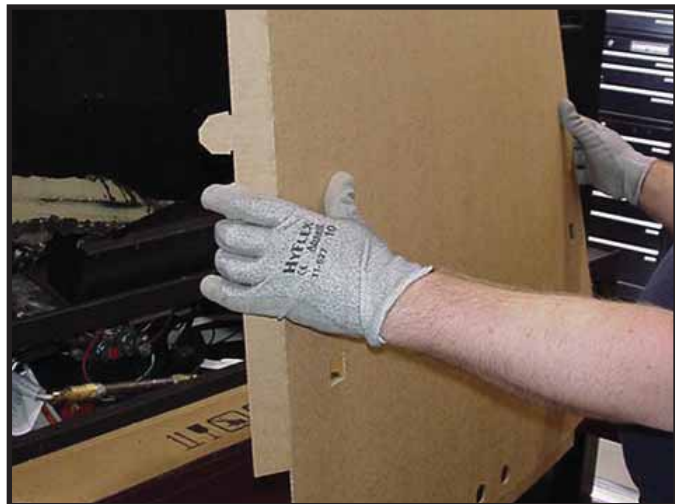
Figure 13.3 Folding of Right and Left Sides of Splatter Guard
