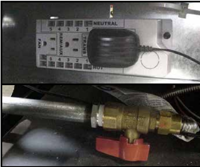
Figure 13.5 Preparation to Install Splatter Guard
