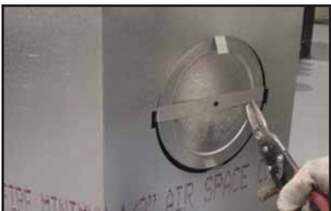
Figure 6.9 Cut the metal retaining band and fold the sides out.
