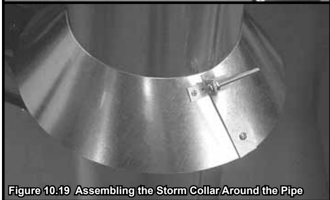
Figure 10.18 Assembling the Storm Collar
