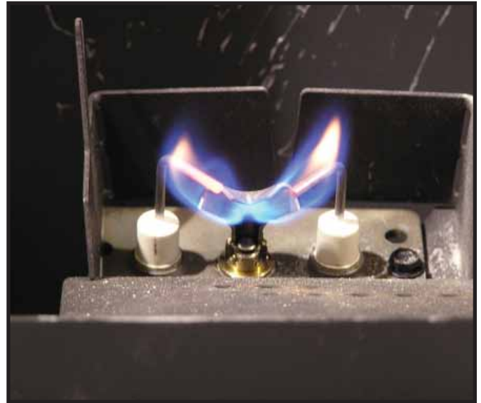
Figure 3.1 IPI Pilot Flame Patterns
