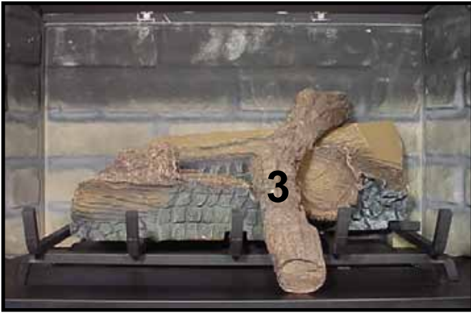
LOG #3 (SRV385-723): Rest log #3 on the grooves on log #1 and log #2.
