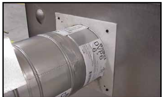
Figure 27. Attach the first flue section (it will snap into place). Slide the insulation gasket onto the flue section, up against the appliance and over the tabs. Use two self-tapping screws to secure gasket to outer wrap.
