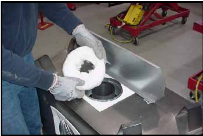
Figure 21. Remove the insulation from the outer flue pipe.
