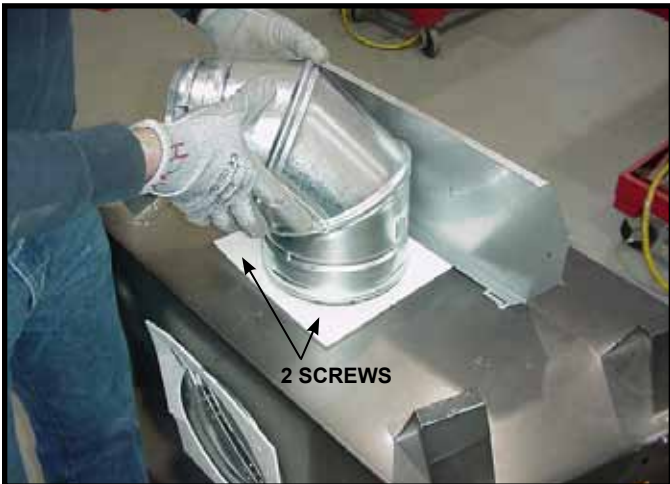
Figure 22. To attach the first section of flue pipe, make sure to use the fiberglass gasket to seal between the first flue pipe component and the outer fireplace wrap. Use 2 self tapping screws to secure the gasket to the outer wrap.
