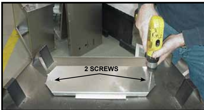
Figure 16. For top flue, remove the two screws holding the top heat shield in place. For rear flue, see next page.
