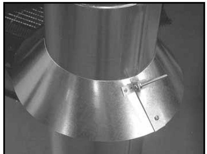
Figure 46 Assembling the Storm Collar Around the Pipe
