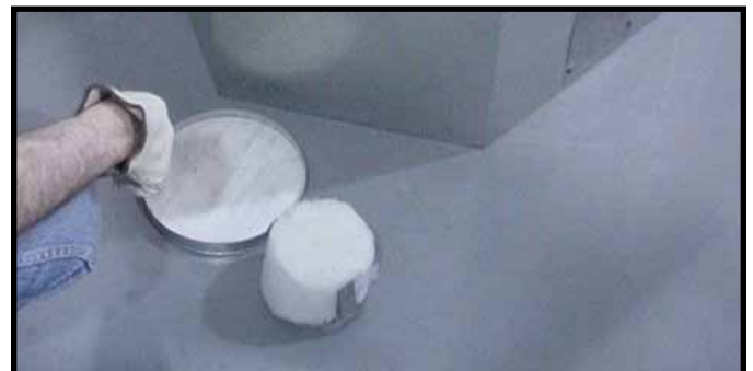
Figure 26. Discard the flue cap, remove and discard the insulation basket. Note: Once the flue cap has been removed it CANNOT be reattached.
