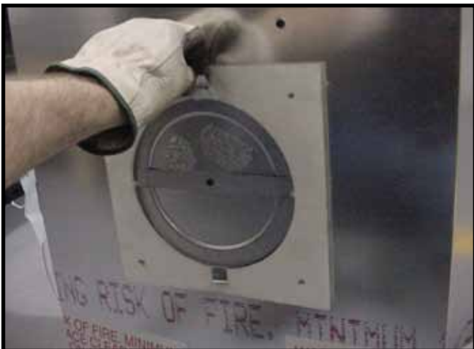
Figure 23. Remove the insulation from the outer flue pipe.
