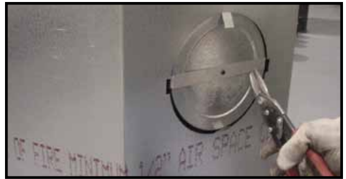
Figure 24. Cut the metal retaining band and fold the sides out.
