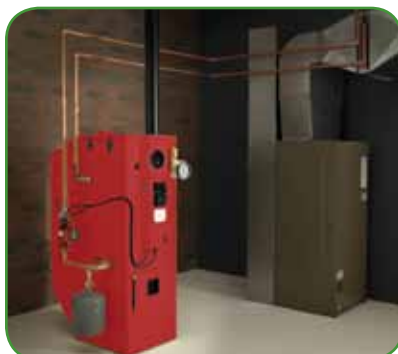
BH60 Pellet Boiler installed with a water-to-air heat exchanger in an existing forced-air furnace.
